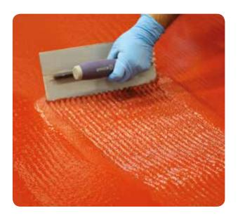
Localised floor movement or existing structural joints can crack even the sturdiest of floor finishes. To solve this, flexible joint solutions can be installed during the application process that protect against damage from these sources.
